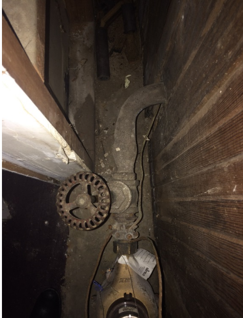
Figure 2: A lead service line
